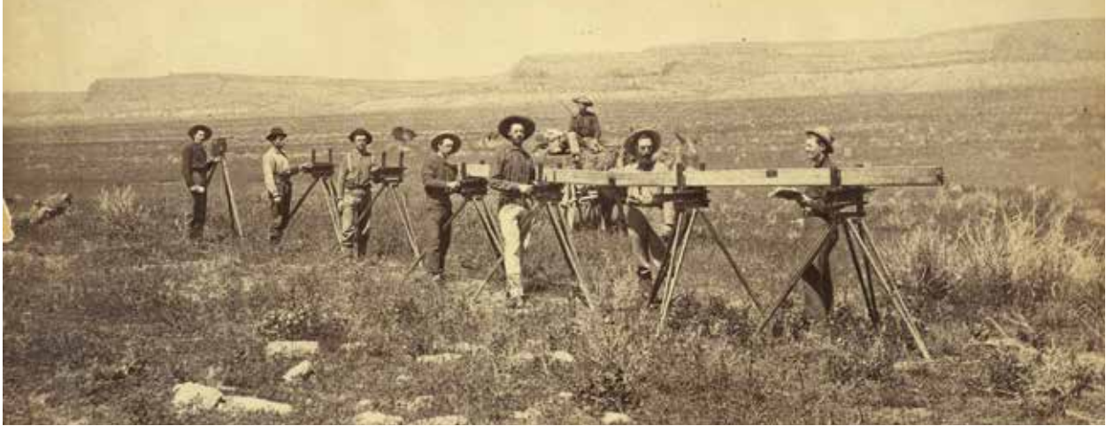
U.S. Geological Surveyors measuring a baseline near Fort Wingate, N.M., in 1883.
